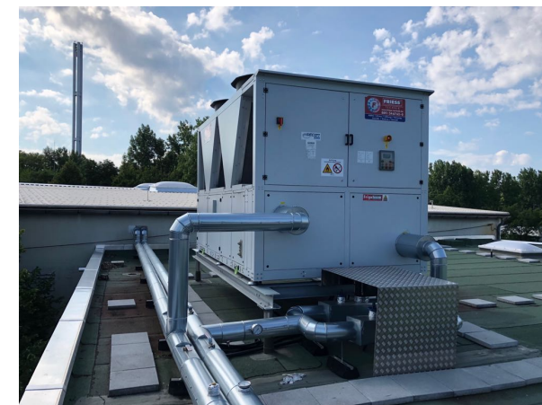
200kW Indirect R290 Chiller (Germany) Total refrigerant utilised: 14 Kg's R290
