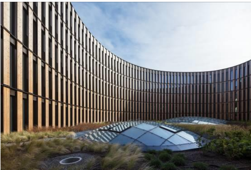
Caption: On the aluminium facade of the Freiburg administrative centre, which is a post-and-bar construction, vertical photovoltaic elements have been placed on surfaces where the sun's rays have been calculated to be optimum.
